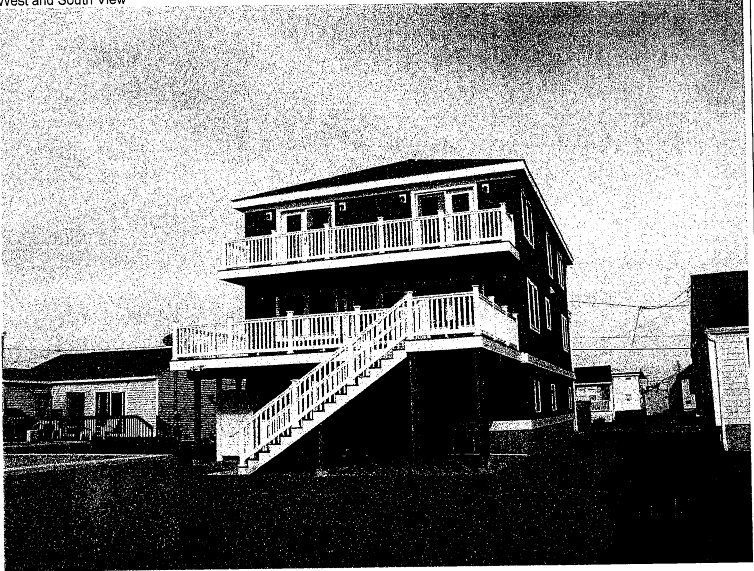
West and South View
