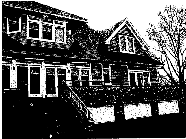
Rear View Breakaway Panels Shown Typical
