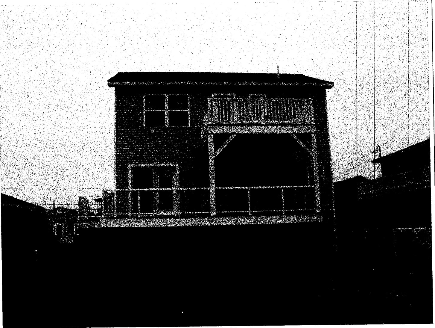
Rear View (East)
